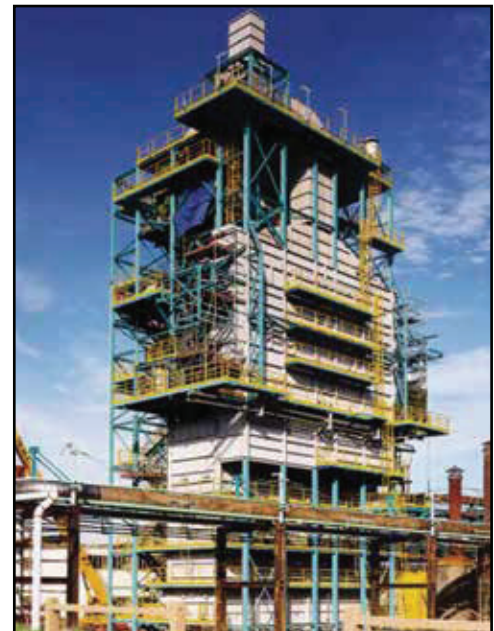
Ethylene Cracker Unit
